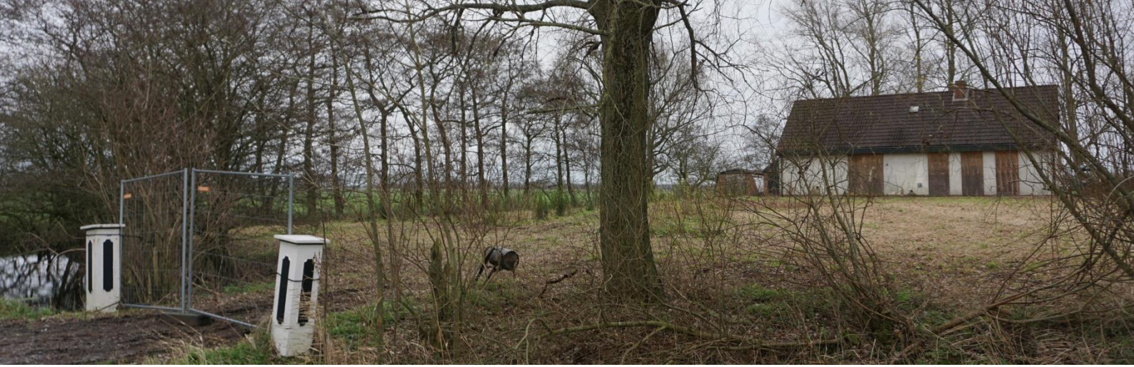
An abandoned house in Loppersum, damaged by mining-induced earthquakes. 11
