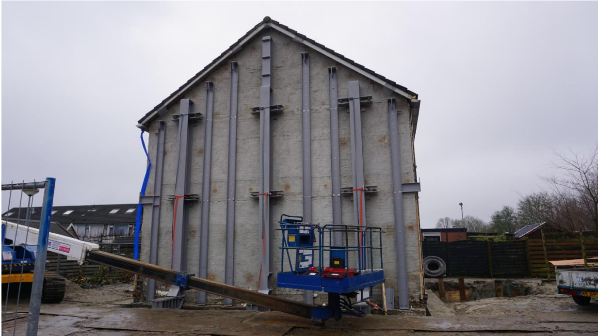
Figure 10: A house that is being reinforced in Opwierde-Zuid.
